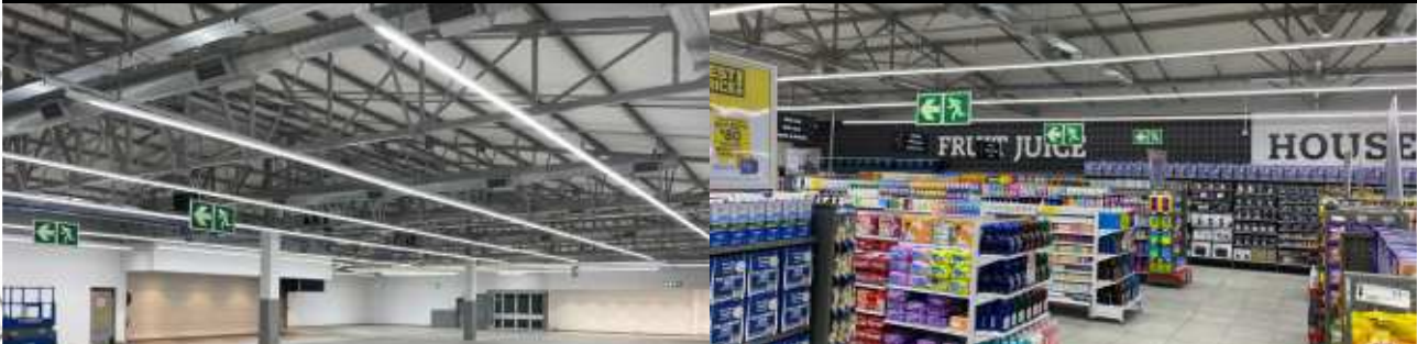
Pnp Pretoria North - Refurbishment
